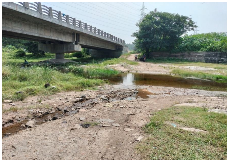
Fig: Korayar at Pudussery
